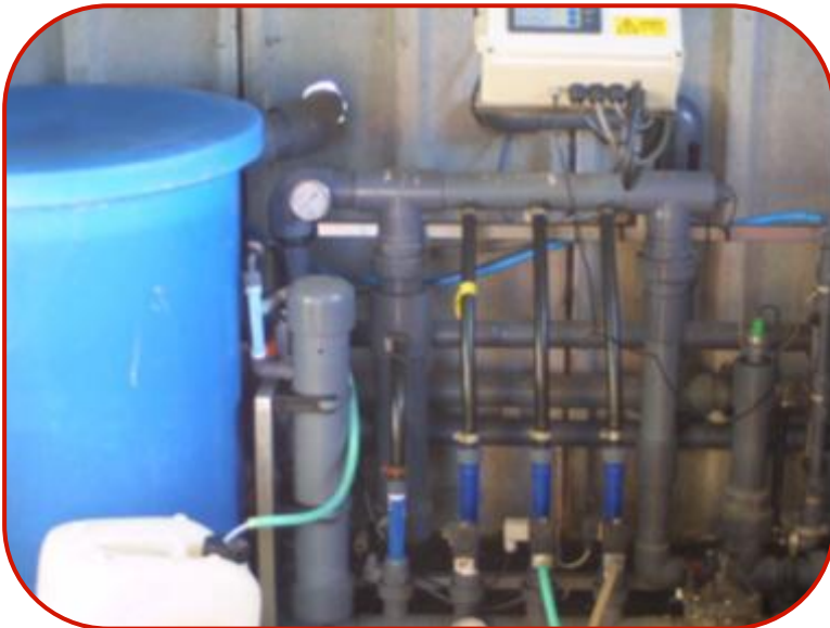
Figure 2.16: The nutrification control unit of the soilless cultivation plot in the UK Source: Atwood et al, 2005
