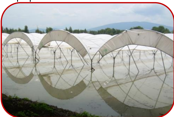
Figure 6.11: A flooded macro-tunnel
